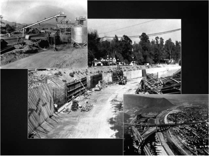
River being concreted
